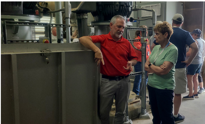
City of Lincoln staff discussed the Lincoln Water 2.0 project at the Ashland wellfield.
